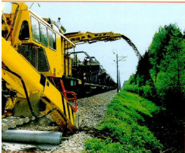
ing the line open, a multi-function machine is used to rebuild the railway bed without
